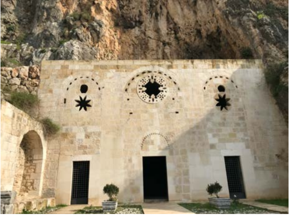
Saint Pierre's Church, Antakya
